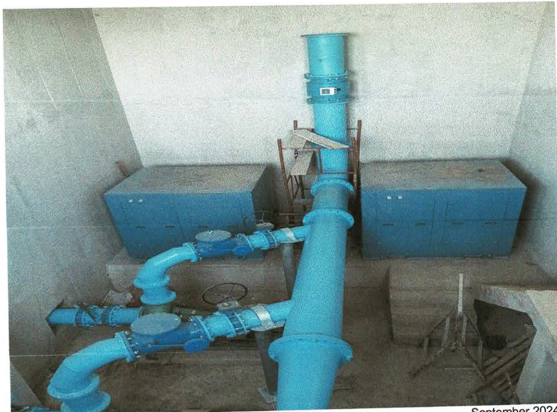
Installation of Backwash Delivery Pipework
