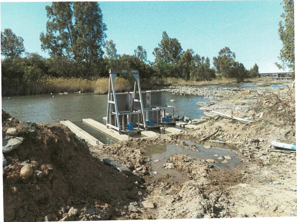
River Chambers: Screen and duck foot alignment
