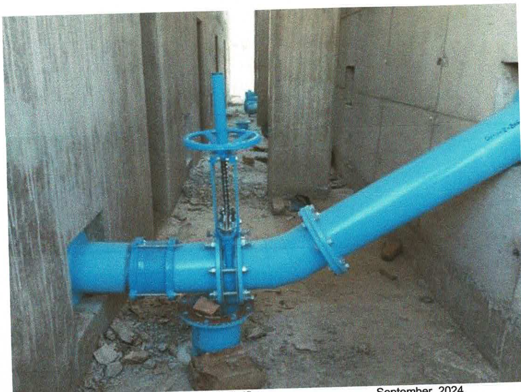
Installation of sludge draw-off pipework at clarifier
