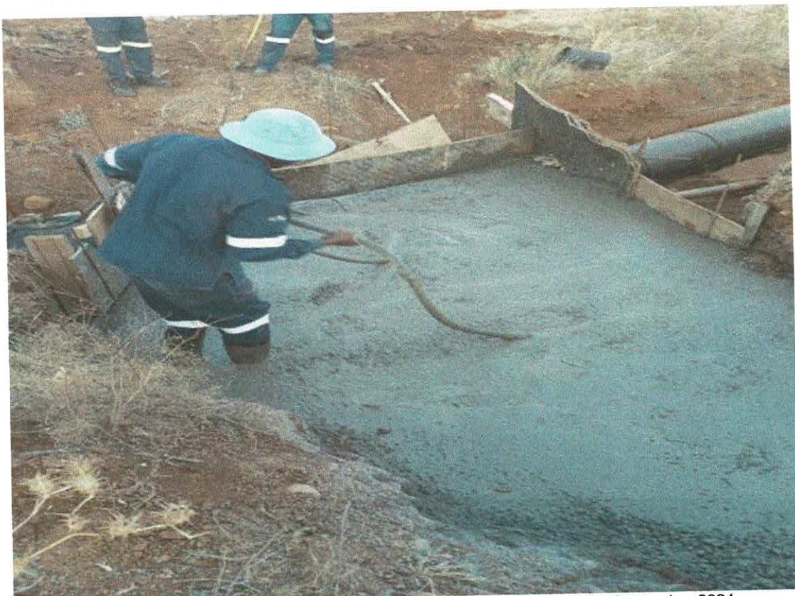
Installation of Thrust Block on Raw Water Pipeline
