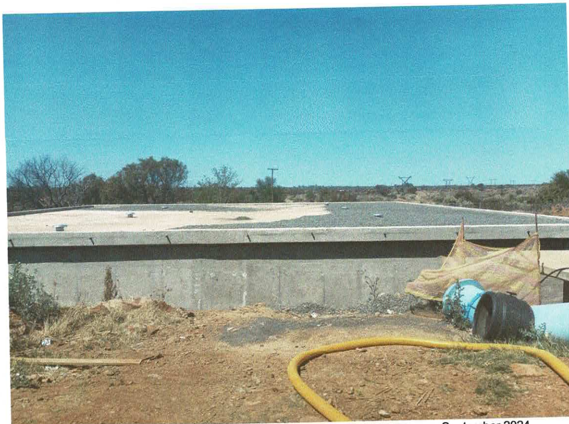
Clear water reservoir: 19mm gravel placement on roof
