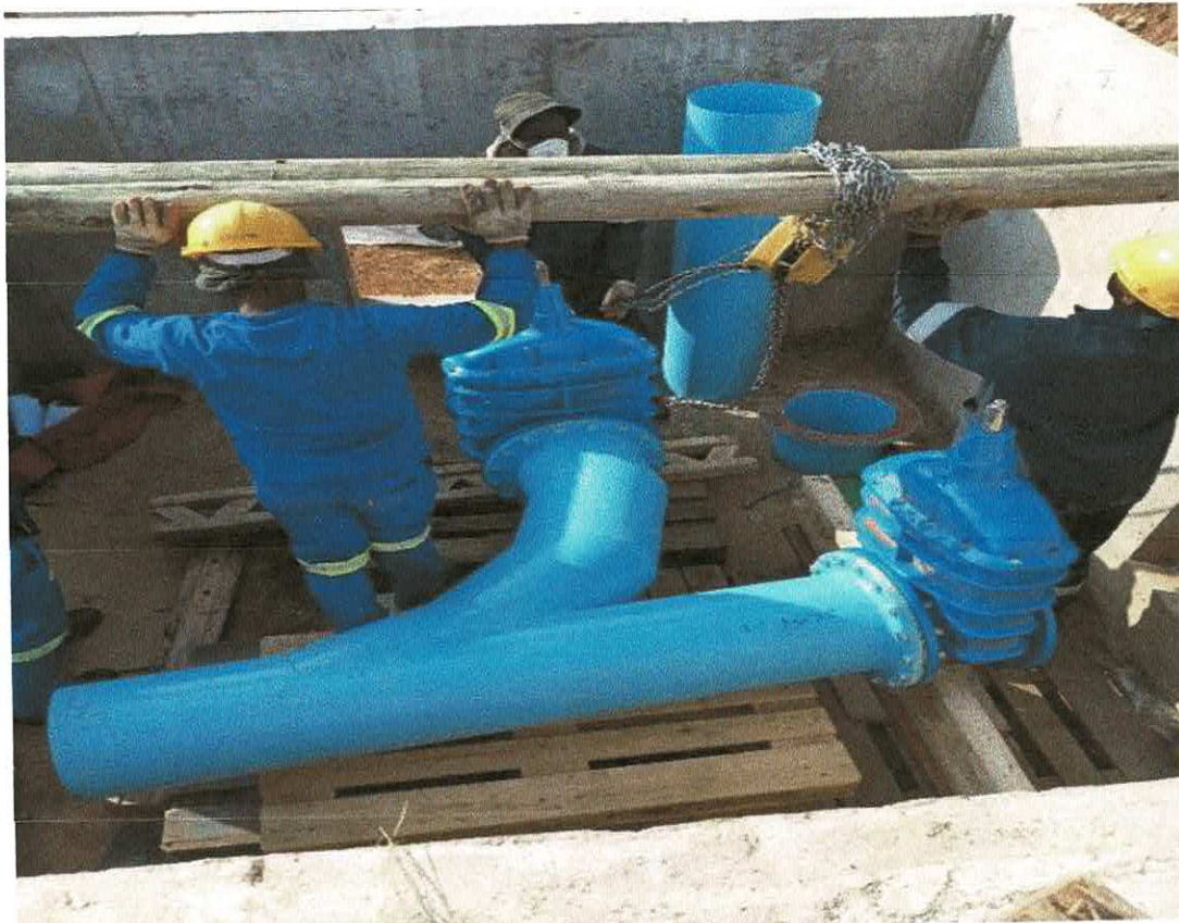
Installation of Pipework in Raw Water Inlet Chamber
