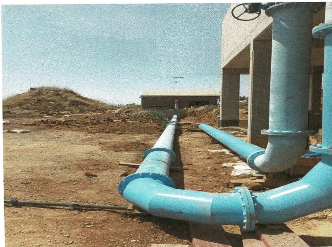
Installation of Pipework at Primary Flocculation
